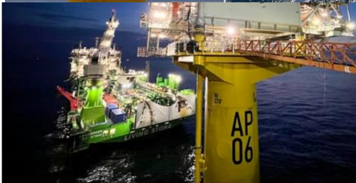
A look at the South Fork Wind substation under construction off the coast of Long Island.
