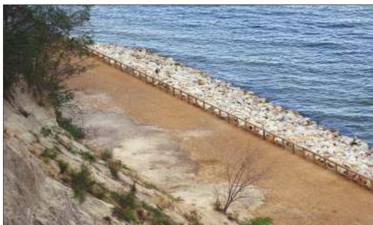
Babie Doly. Opaska brzegowa u stopy klifu. The seawall in Babie Doly at the bottom of the cliff.
