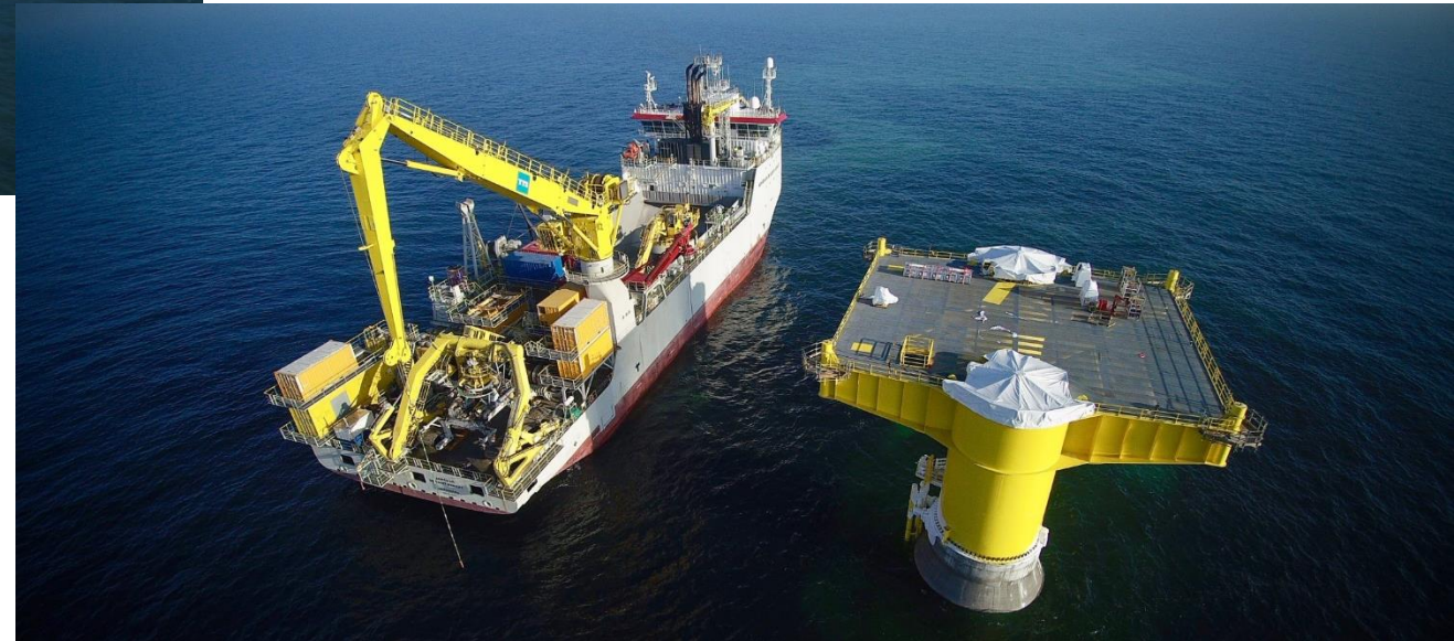
Denmark – Kriegers Flak Offshore Sub-Stations - Design, Construction, Transport and Installation of 2 Gravity Based Structure Foundations - FPV Adhémar de Saint-Venant
