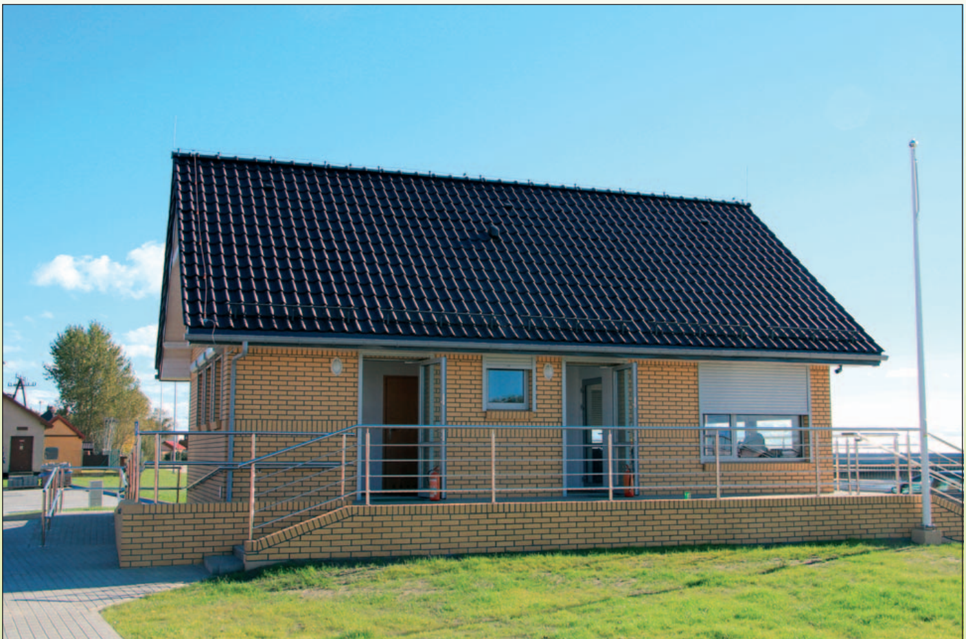
Ukończony budynek bosmanatu. Z archiwum UM w Gdyni. The finished building of the bosun's office. Photo by courtesy of Gdynia Maritime Office. Das fertige Bootsmann-Amt. Foto aus dem Archiv des Seeamtes Gdynia.
