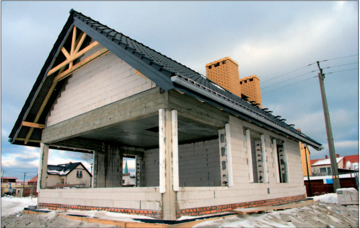
Luty 2012 – stan surowy budynku bosmanatu. Z archiwum UM w Gdyni. February 2012 – Unfinished bosun's office building. Photo by courtesy of Gdynia Maritime Office. Februar 2012 – Rohzustand des Bootsmann-Amts. Foto aus dem Archiv des Seeamtes Gdynia.
