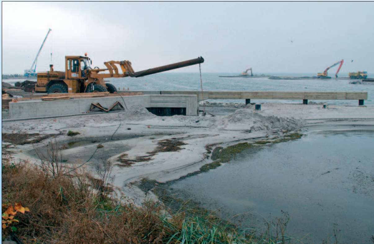
Listopad 2011 – żelbetowe elementy nowego slipu. Z archiwum UM w Gdyni. November 2011 – Reinforced concrete elements of the new slipway. Photo by courtesy of Gdynia Maritime Office. November 2011 – Stahlbeton Elemente des neuen Hellings. Foto aus dem Archiv des Seeamtes Gdynia.
