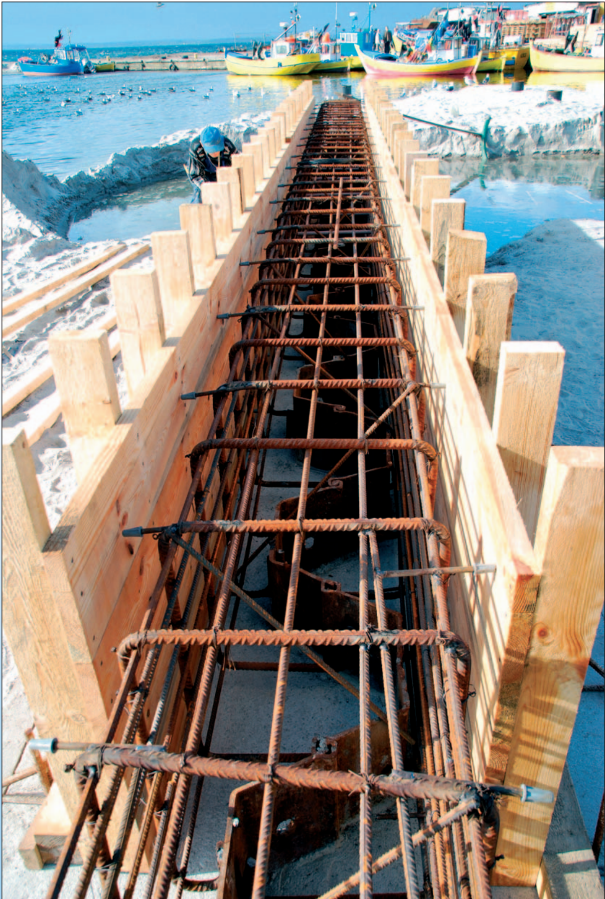
Szalunki oczepów na nowym slipie. Z archiwum UM w Gdyni. Shoring the caps on the new slipway. Photo by courtesy of Gdynia Maritime Office. Verschallungen am neuen Slip. Foto aus dem Archiv des Seeamtes Gdynia.
