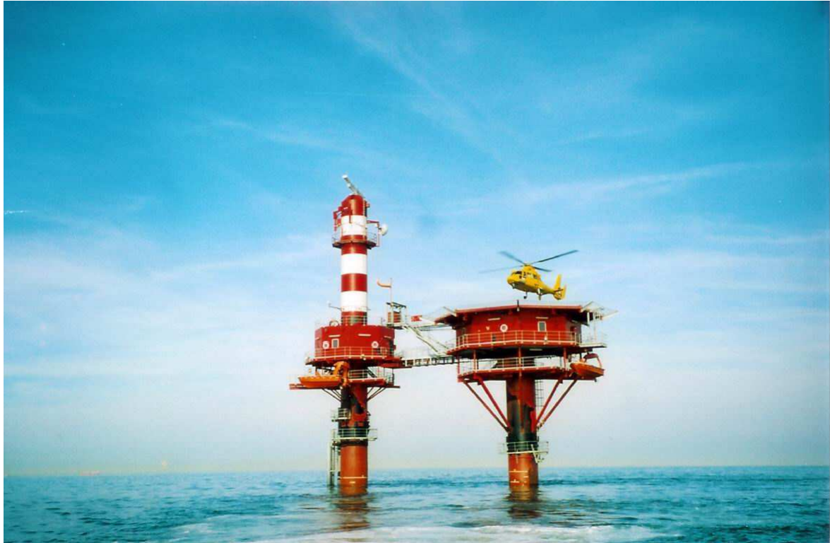
Radar is a key requirement for most VTS. Siting the antenna in the right location and obtaining adequate height requires much consideration. Some solutions: above, an automatic facility at Oostdyckbank, ten miles off the Belgian coast (Flemish Waterways); below left, at Saeftinghe, and below right, the old tower a La Maddalena, Italy. (Italian Coastguard)
